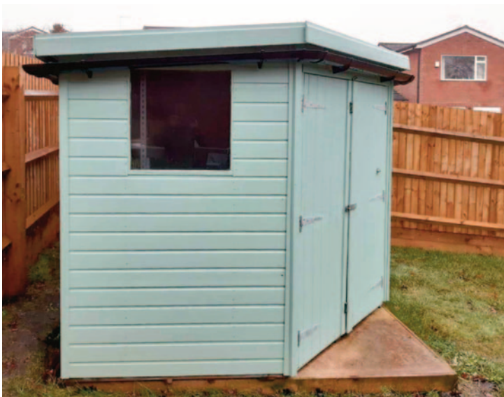
Protected with Protek Royal Exterior. All corners, glass, and doors sealed with mastic and silicon. Gutters fitted on all four sides.
