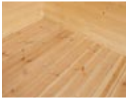
FLOOR: 28mm tongue and groove floor.
